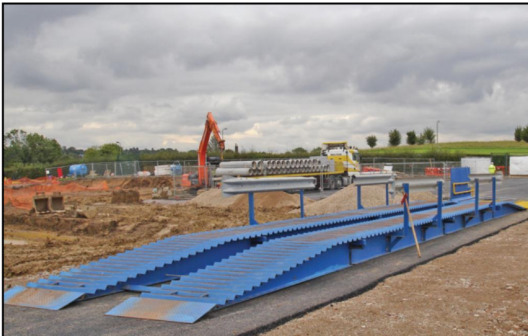
Figure 4-2 Typical wheel wash using the dry ramp system
