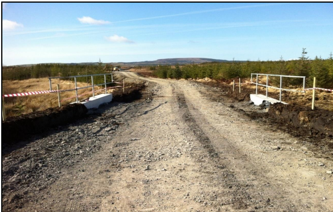
Figure 48: Dirty water containment at watercourse crossings
