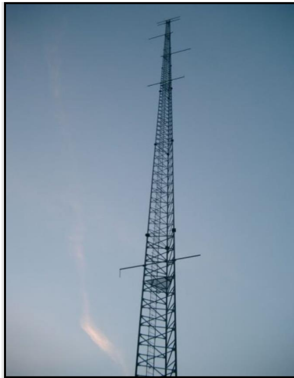
Figure 16: Typical meteorological mast on a wind farm
