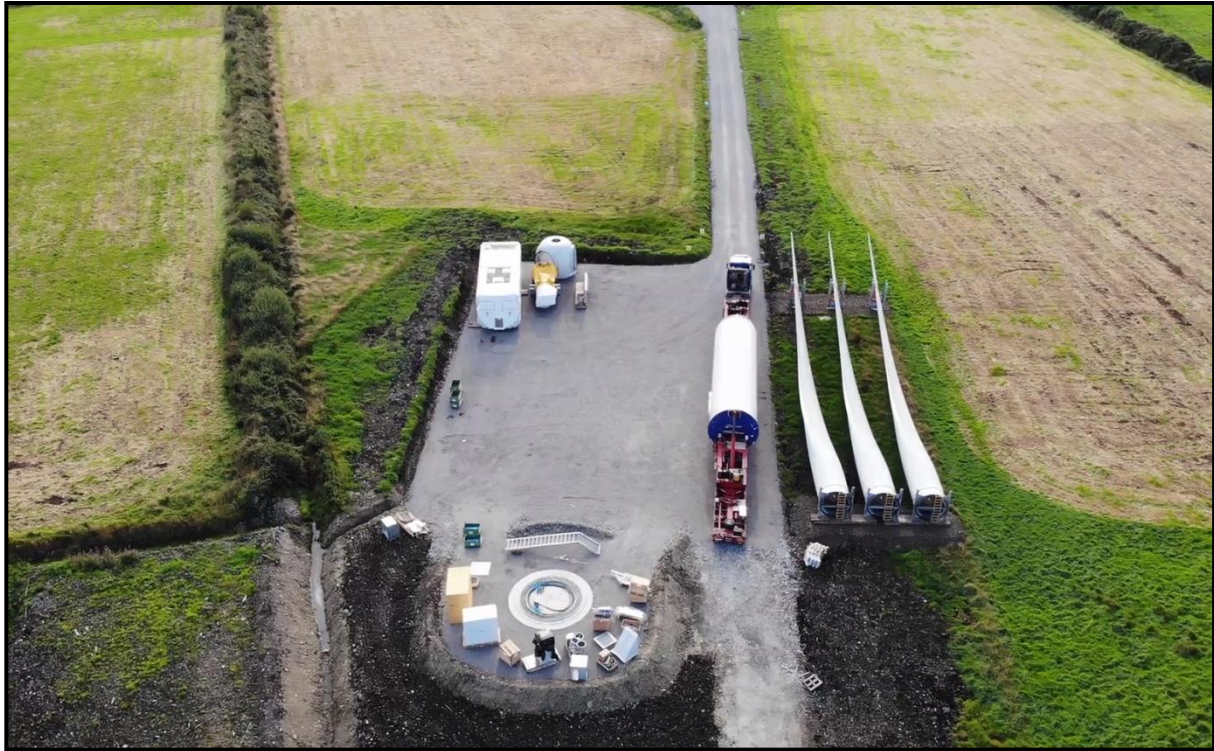
Figure 4.7 Typical finished hardstand on a wind farm
