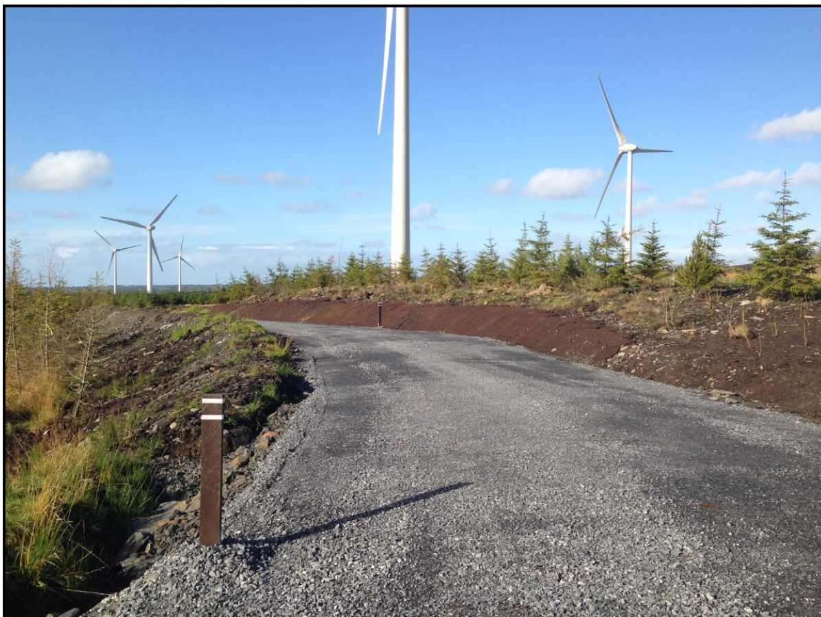
Figure 20: Typical new excavated road on a wind farm
