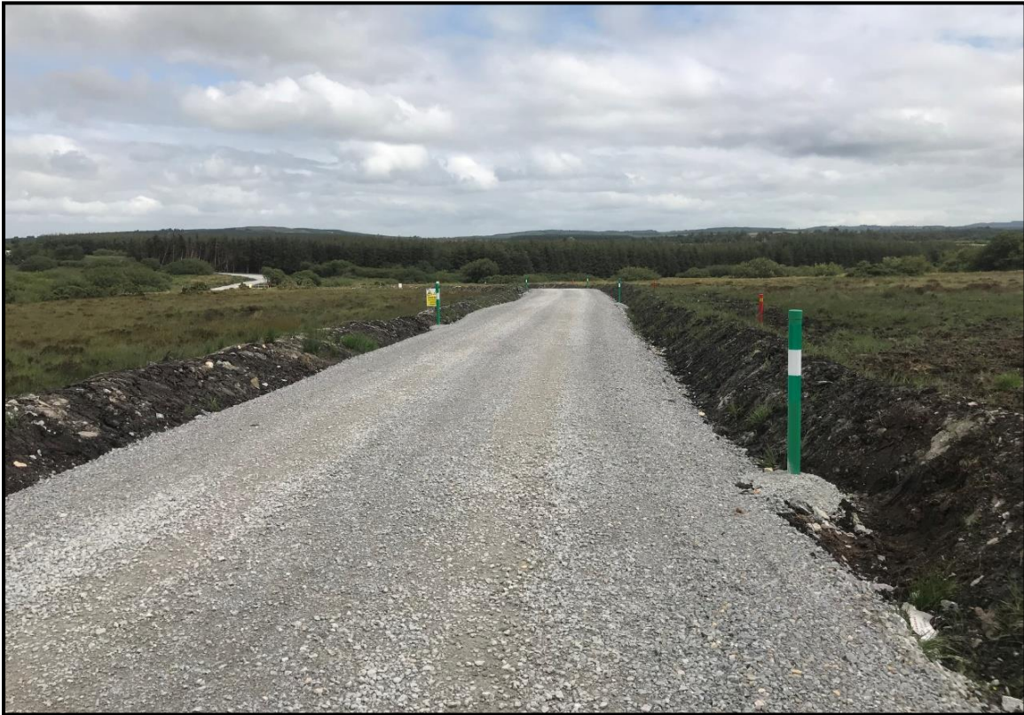
Figure 21: Typical floated road on a wind farm
