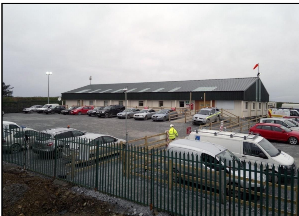
Figure 6: Typical temporary site construction compound on a wind farm
