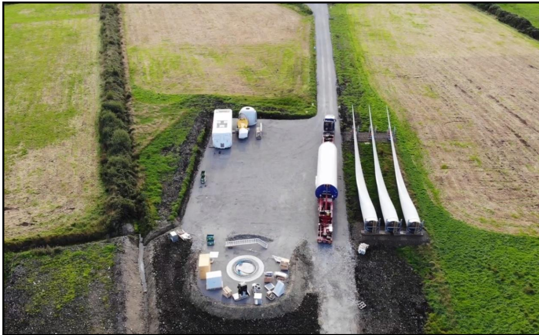
Figure 8: Typical Turbine Hardstand and lay down area
