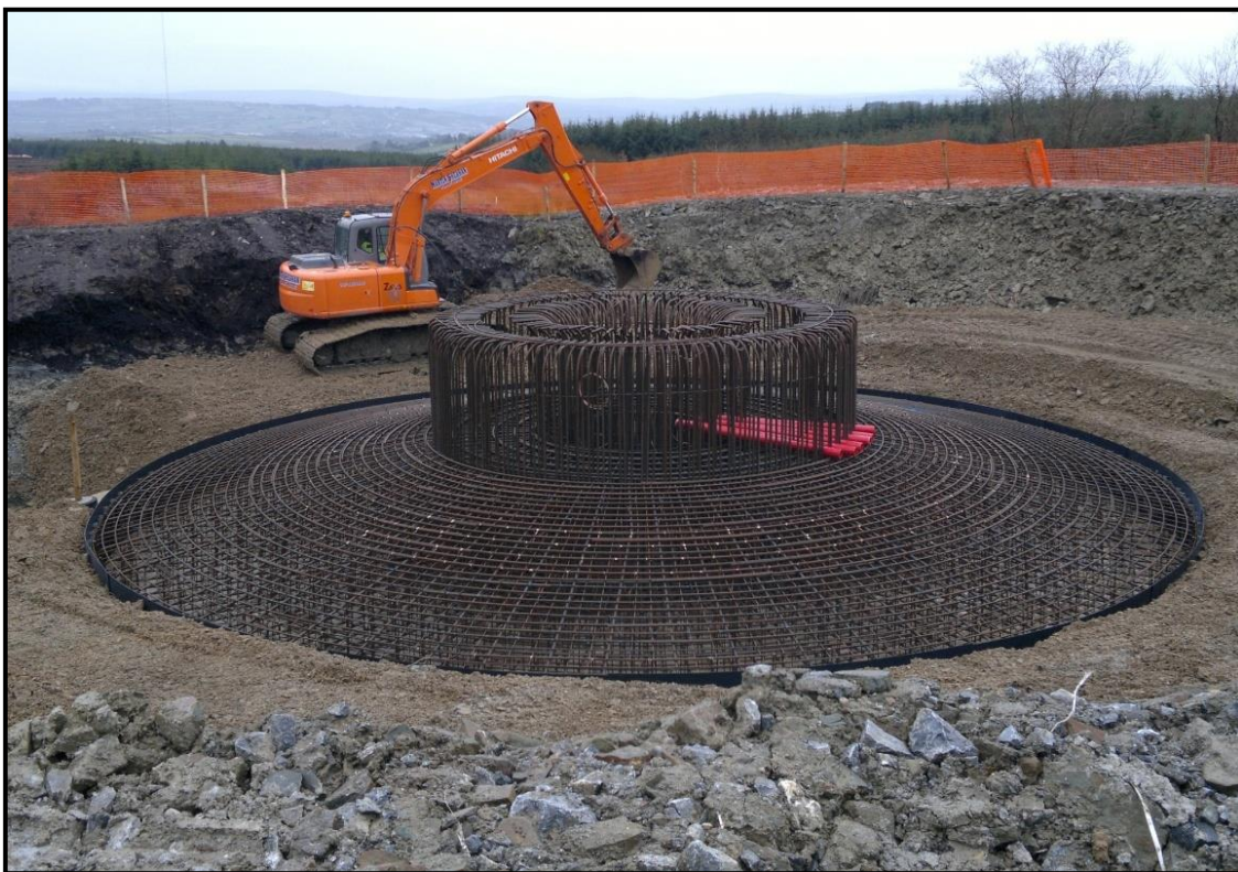
Figure 7: Typical construction of a wind turbine base
