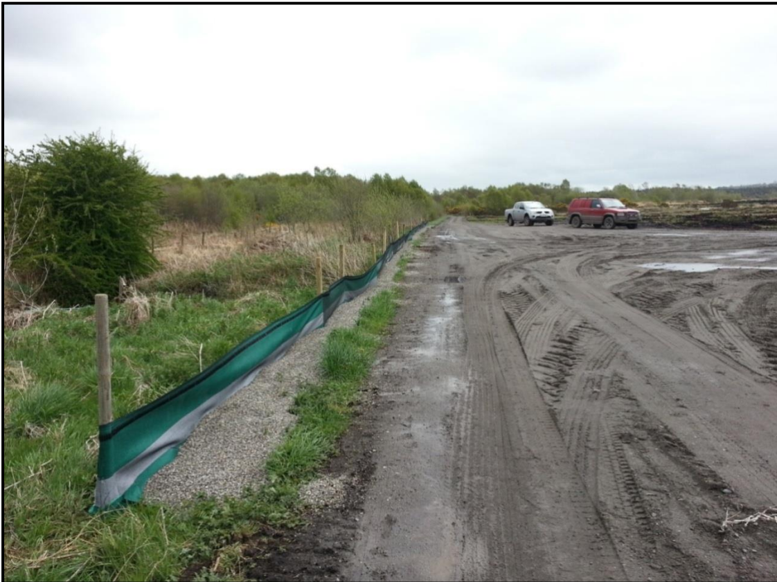
Figure 49: Silt curtain containment along existing roads near watercourses
