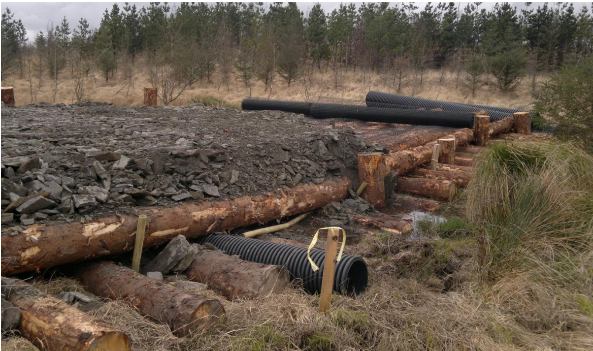
Figure 23: Lightweight floated road in place across flush area
