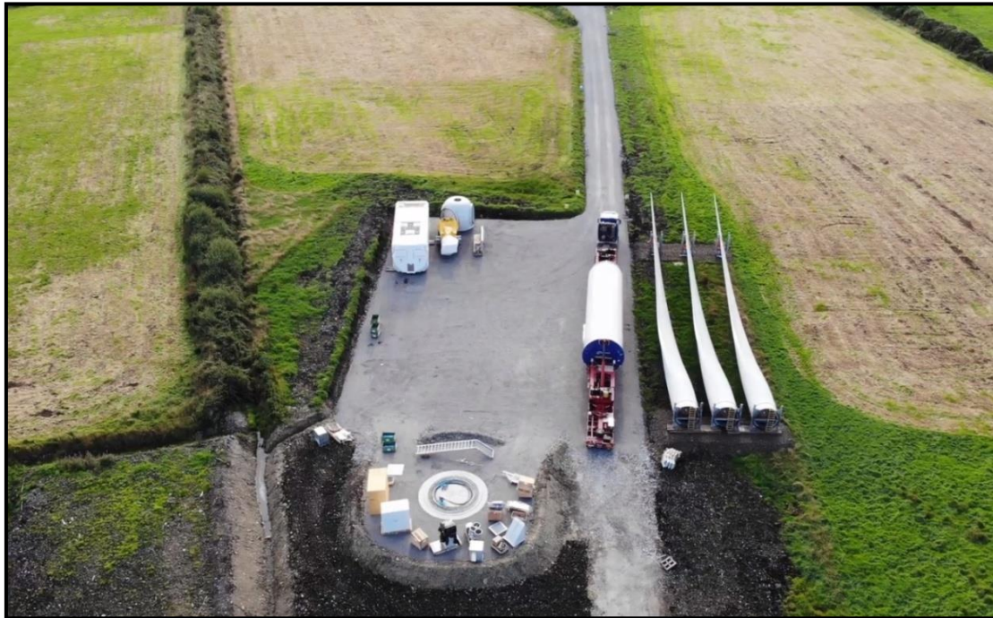
Figure 8: Typical Turbine Hardstand and lay down area
