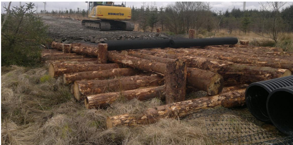
Figure 22: Typical Log Road in process of construction on a wind farm
