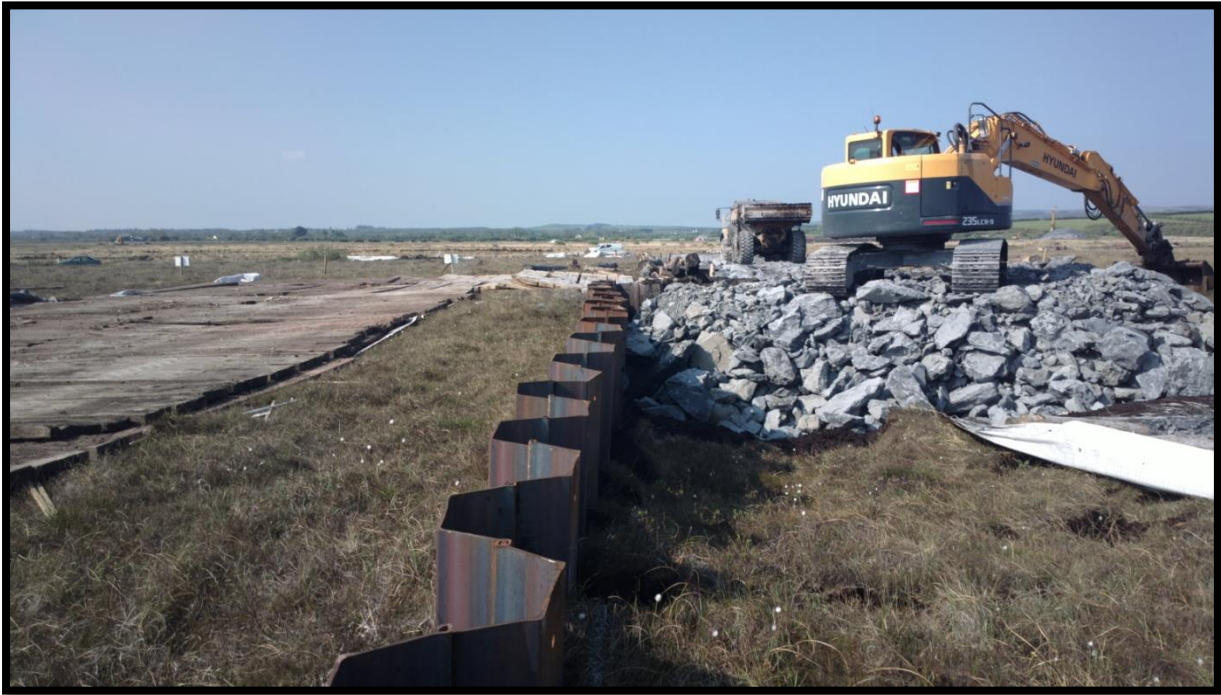
Figure 13: Excavating beside the Sheet Pile Cofferdam
