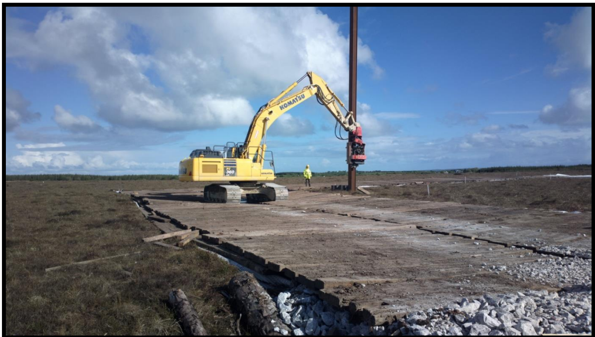
Figure 12: Sheet Pile Installation
