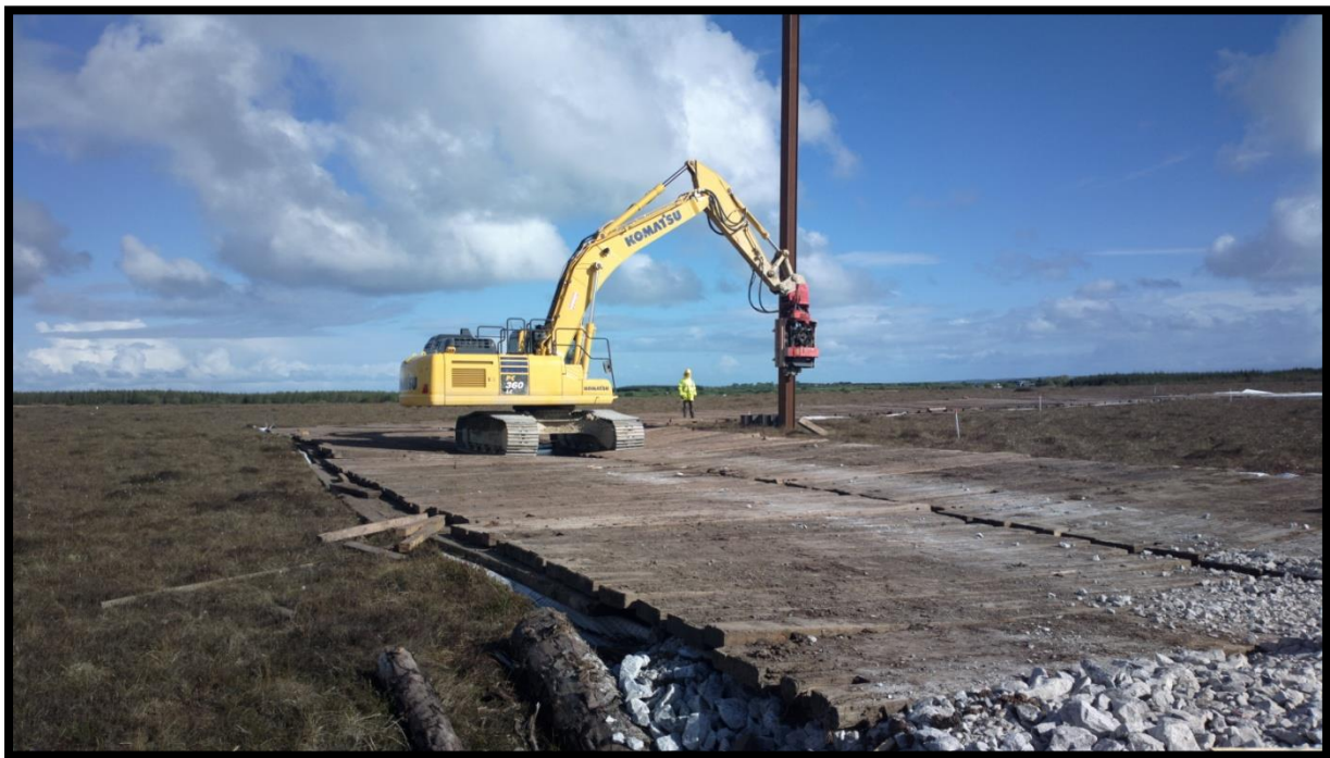
Figure 12: Sheet Pile Installation
