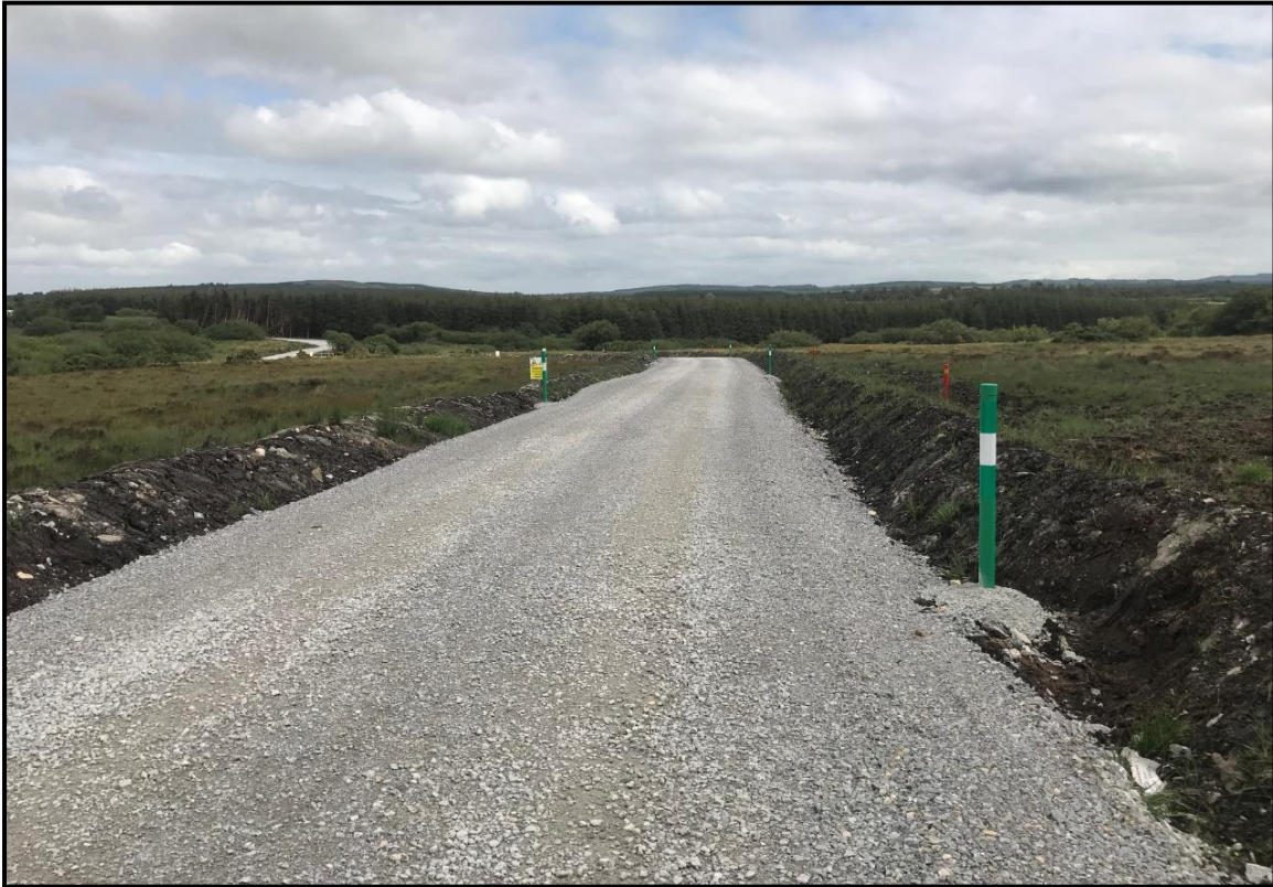
Figure 21: Typical floated road on a wind farm
