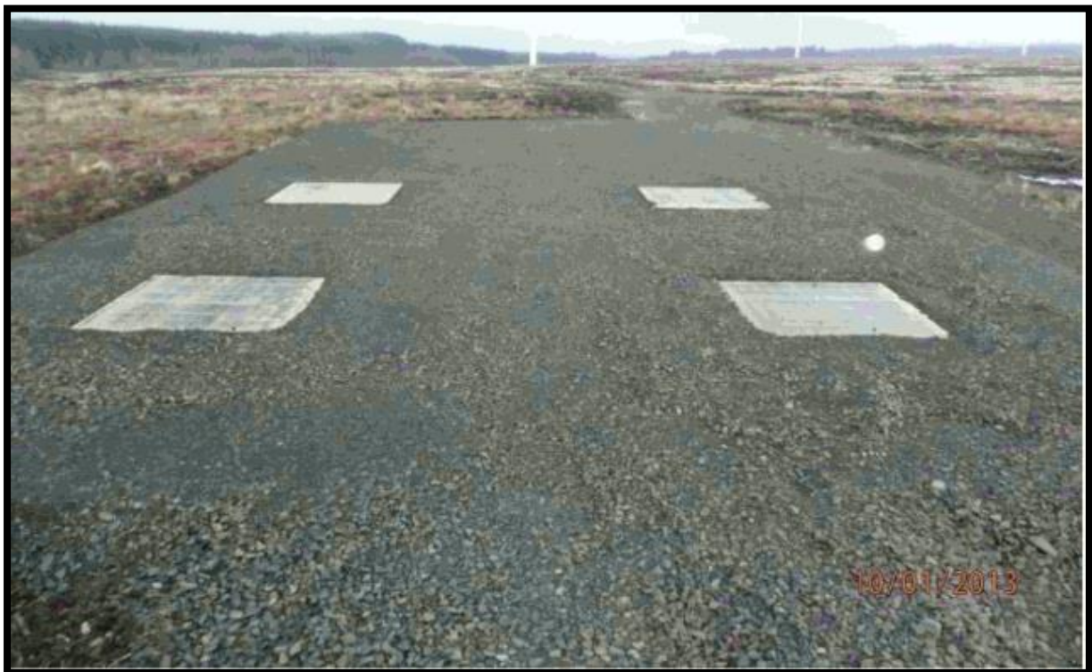
Figure 15: Typical Floating/Piled Hardstand Option
