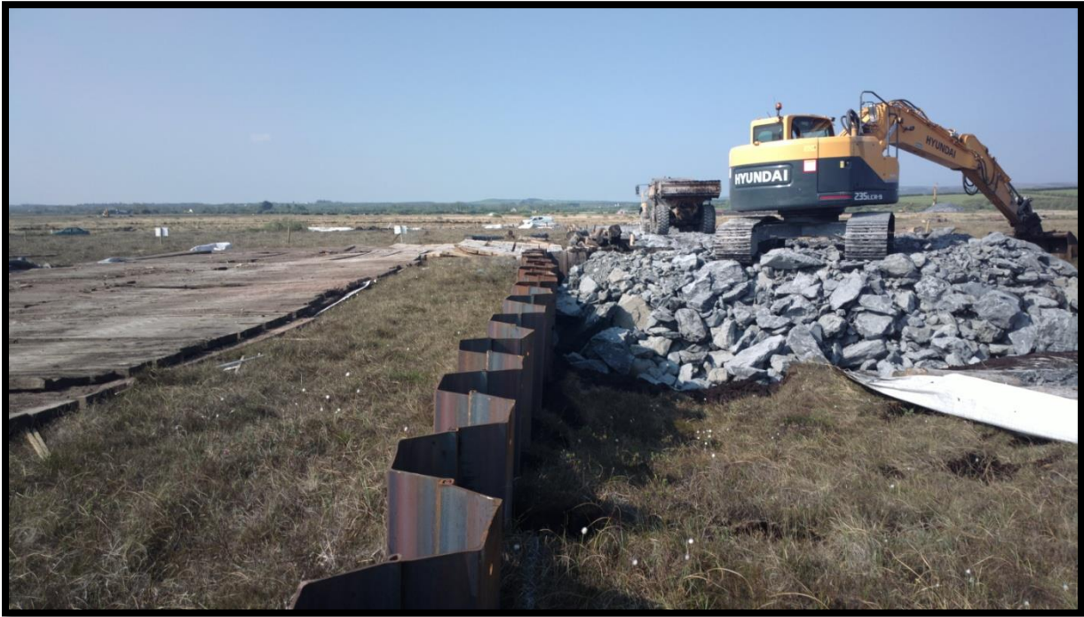
Figure 13: Excavating beside the Sheet Pile Cofferdam
