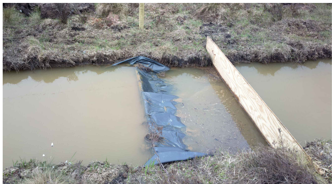
Baffle/Weir Detail
