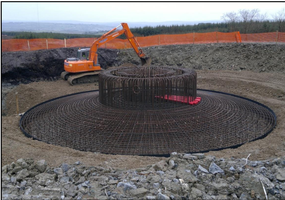
Figure 7: Typical construction of a wind turbine base
