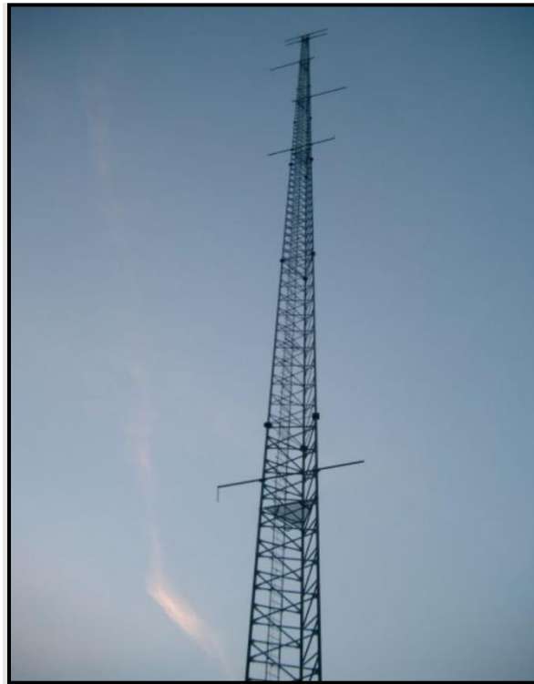
Figure 16: Typical meteorological mast on a wind farm
