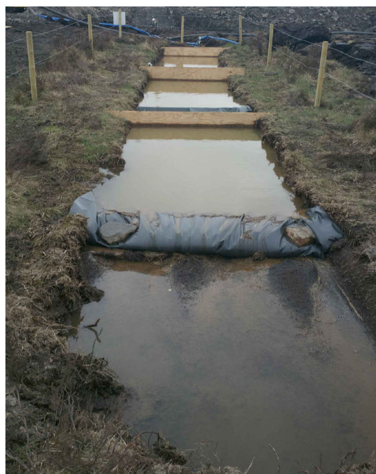
Completed Settling Pond System
