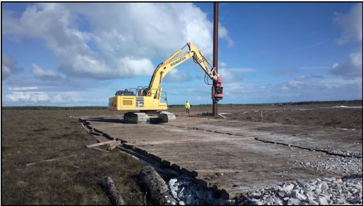
Figure 4-9 Sheet Pile Installation
