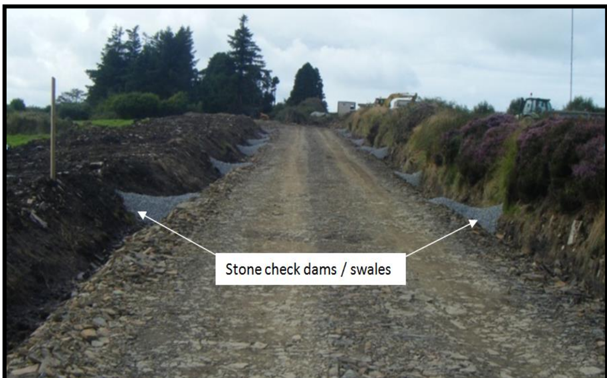
Figure 45: Examples of check dams along roadside drainage channels
