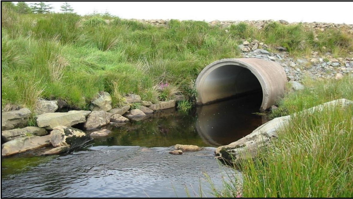
Figure 24: Typical drainage channel crossing
