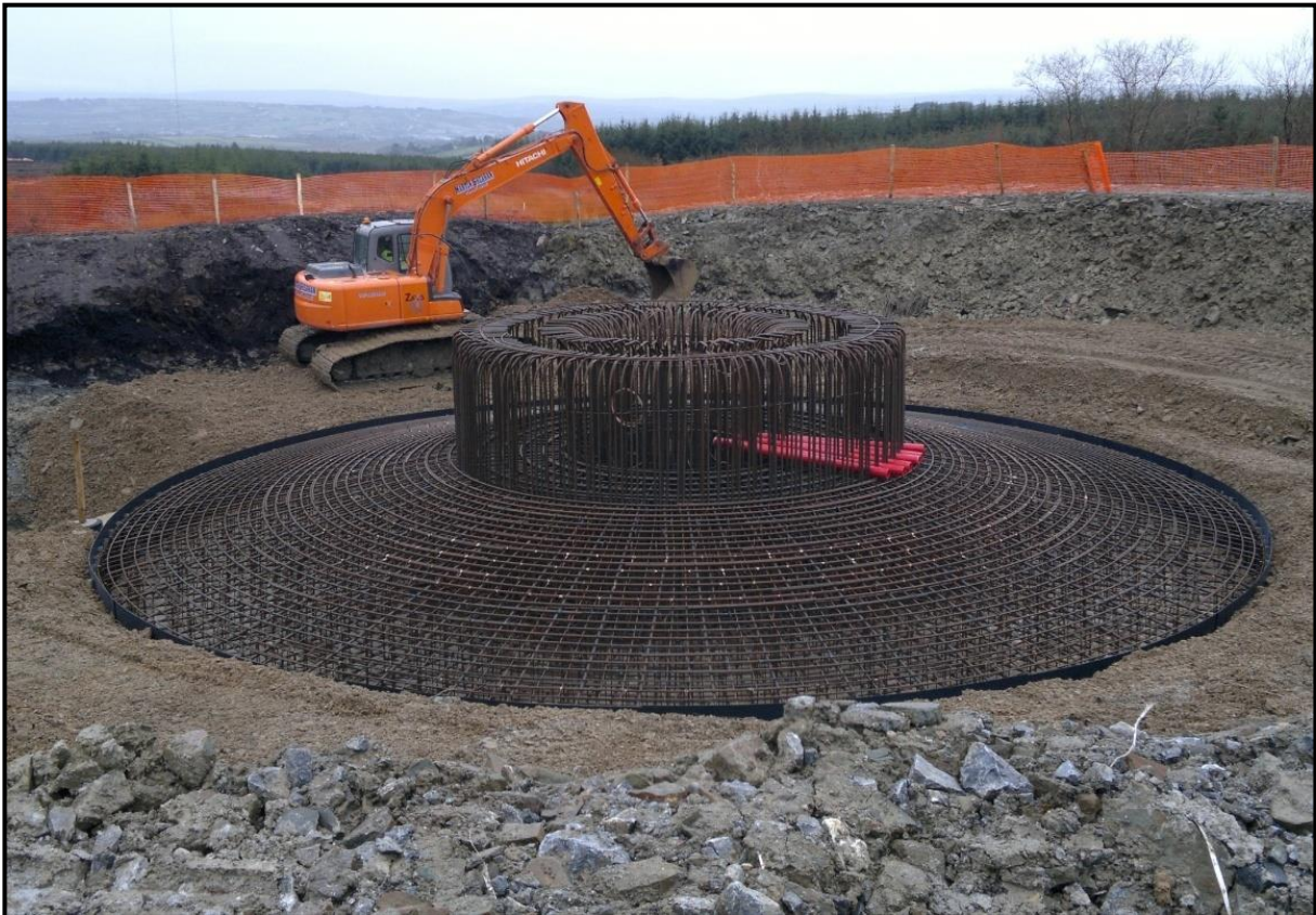
Figure 4.13 Typical construction of a wind turbine base
