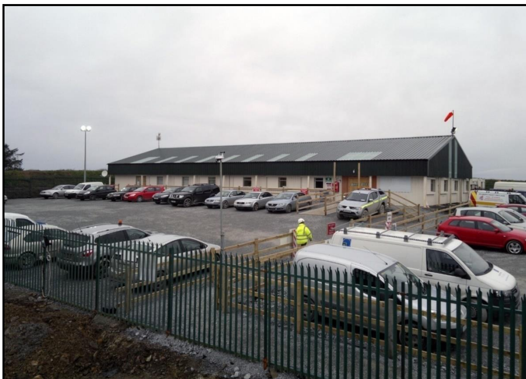
Figure 6: Typical temporary site construction compound on a wind farm
